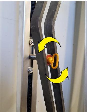
Using the yellow ring provided, turn the manual release rod anti-clockwise, this will unwind the manual release rod from the automatic operator drive carriage. Continue to turn the manual release rod until it come free from the automatic operator drive carriage.
