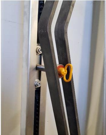
Locate the yellow ring handle manual release turn rod which is positioned between the two steel ramp rails. Ramp rails are located on the same side of the motor and are attached to the back of the door panel.
