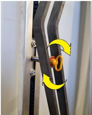
To reconnect the automatic operator to the garage door, manually operate the garage door by hand until the automatic operator carriage lines-up with the steel ramp rails.
